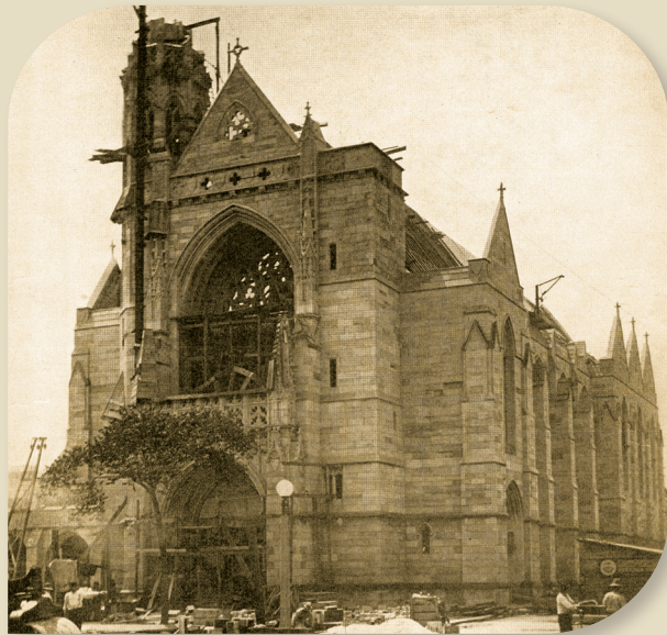
Fourth Presbyterian Church under construction, August 1913
